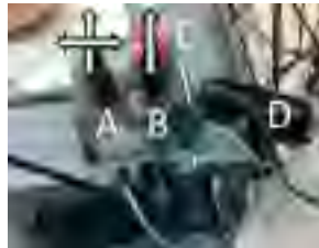
Existing control levers
