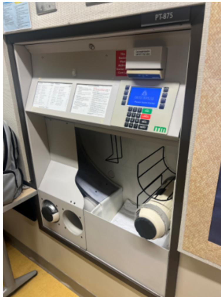
Figure 5: PICU Pneumatic Tube Station No. 845
